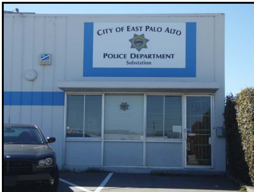
Police Department Parole Re-Entry Substation
