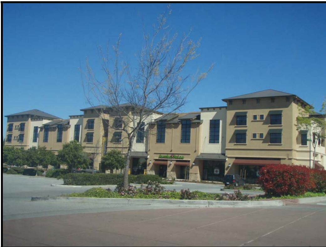
Cummings Park Lofts and Townhomes
