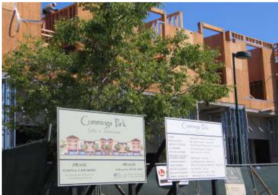
Construction on Cummings Park Lofts and Townhomes
